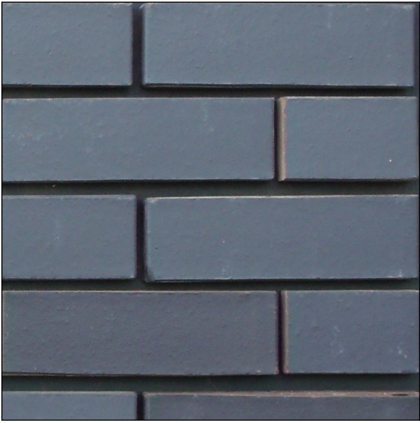
1. Plinth Brickwork (engineering blue)
